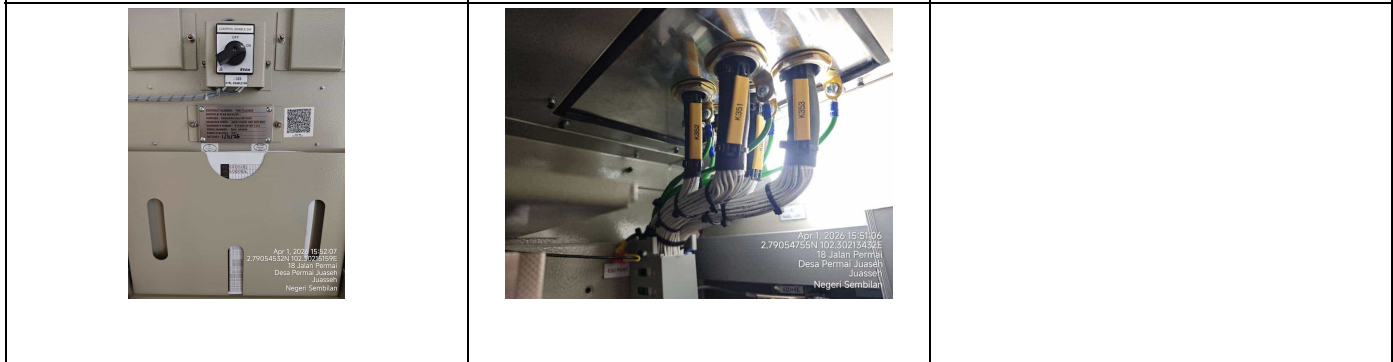
OVERALL PICTURE OF MASTERSHEET INSIDE RTU PANEL CABLES GLAND INSIDE RTU PANEL CABLES GLAND INSIDE RTU PANEL SECOND PIC (IF ANY)
