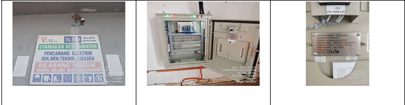
OVERALL PICTURE OF SUBSTATION OUTER WALL (WITH SUBSTATION NAME) RTU AFTER INSTALLATION (WITH INSIDE PICTURE) RTU WARRANTY STICKER (COMPLETE WITH SAT DATE)
