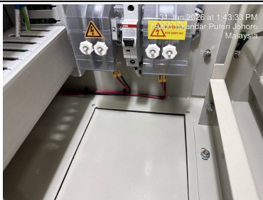
RTU AFTER INSTALLATION
