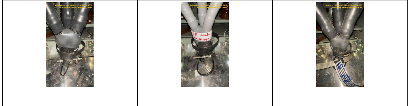
SAMPLE EFI'S CT CABLE AT SWITCHGEAR (AFTER CLAMPED) SAMPLE EFI'S CT CABLE AT SWITCHGEAR (AFTER CLAMPED) SECOND PICTURE (IF ANY) SAMPLE EFI'S CT CABLE AT SWITCHGEAR (AFTER CLAMPED) THIRD PICTURE (IF ANY)
