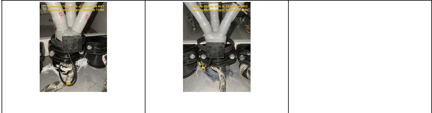
SAMPLE EFI'S CT CABLE AT SWITCHGEAR (AFTER CLAMPED) SAMPLE EFI'S CT CABLE AT SWITCHGEAR (AFTER CLAMPED) SECOND PICTURE (IF ANY) SAMPLE EFI'S CT CABLE AT SWITCHGEAR (AFTER CLAMPED) THIRD PICTURE (IF ANY)
